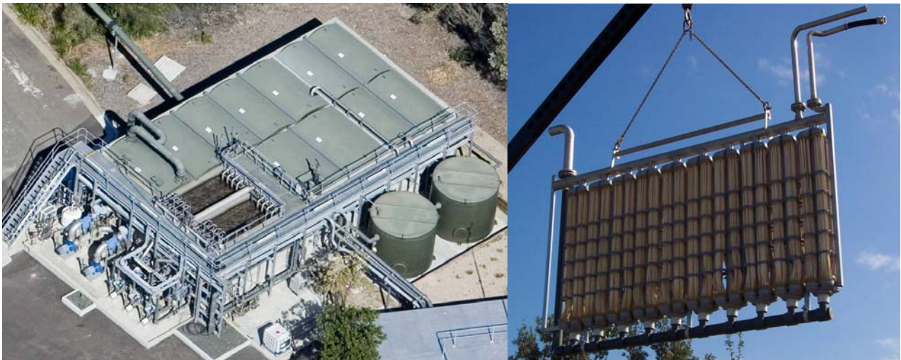
Picture of the North Head's MBR plant (Courtesy of Sydney Water)
