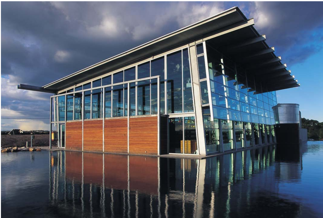
Picture of the Sydney Olympic Park's Water Reclamation Plant (Courtesy of SOPA).
